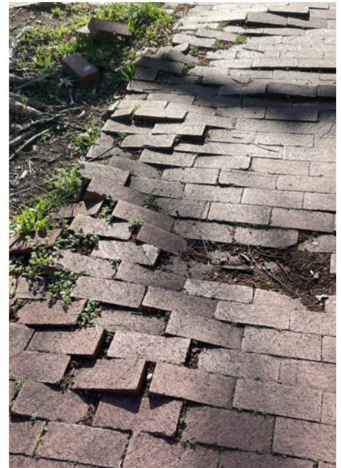
Typical damage to brick sidewalks found throughout Capitol Hill. Navigating these surfaces when you have mobility or balance issues is very difficult and dangerous.
